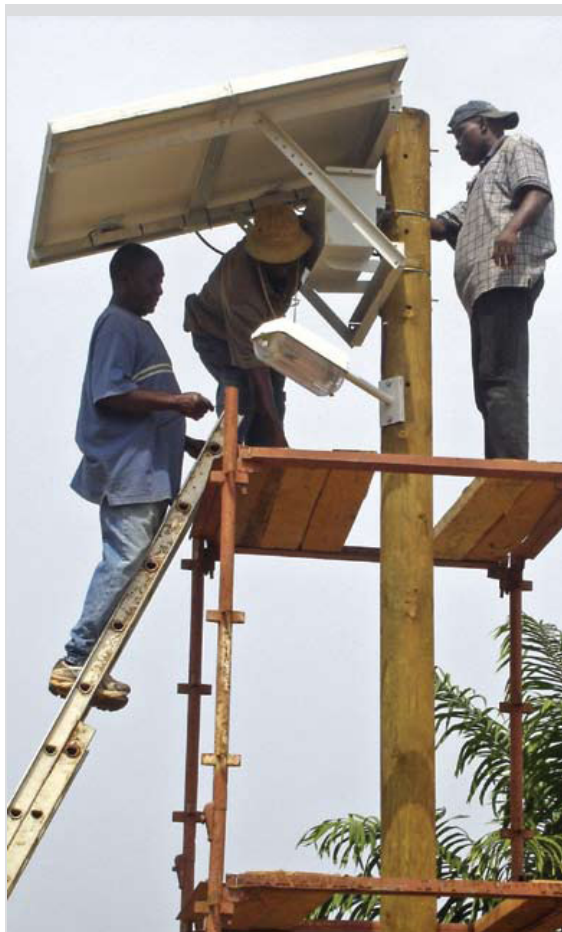
Workers install a solar-powered street light in Robertsport. Solar light panels are attached to sturdy aluminum mounting racks, each including a maintenance-free battery and a “dusk to dawn” charge controller.
