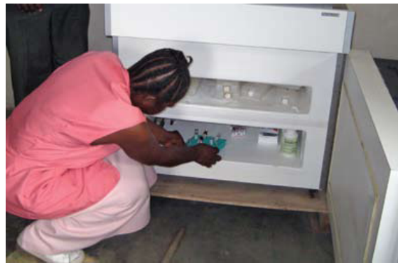
A solar-powered vaccine refrigerator keeps medicines cool.
