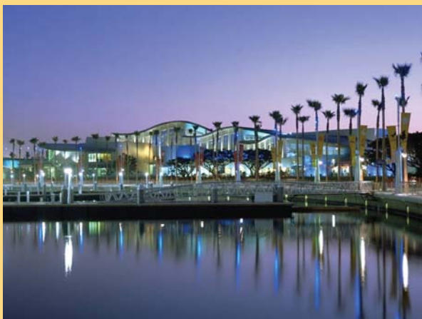
Energy costs are the Aquarium's second largest expense
