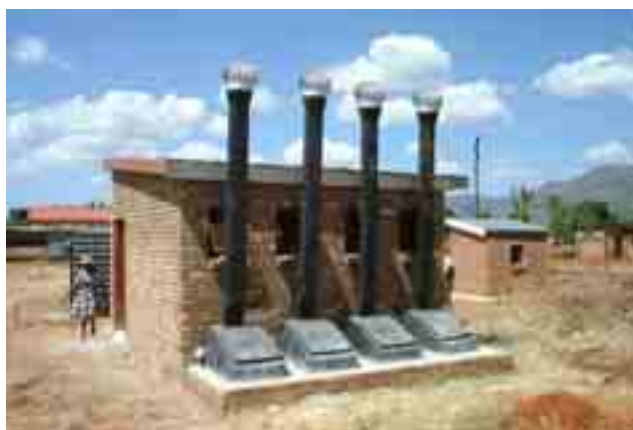
Exhibit 20. Students at one ENCAP EA course reviewed these "enviroloo" (dry composting toilets) mandated by the Department of Public Works in the Northern Province of South Africa.
