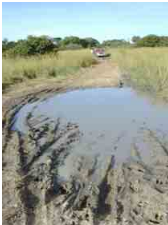
Exhibit 23. A farm-to-market road near Chibombo, Zambia. Upgrading this road to an all-weather road will require elevating the existing roadbed across a wetland area. Doing so could adversely affect wetland hydrology.
