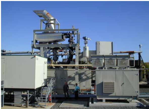
Figure 3. EDL Carbureted Gas Turbine Installation
